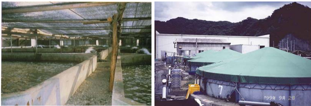
Fig. 2 Typical land-based flounder farms in Japan. Left: square shaped fish tanks made of concrete are installed in shade cloth house; corners of the tanks are rounded off to avoid stagnant water. Right: round shaped fish tanks made of fiberglass reinforced plastic; top of the tank is covered by vinyl sheet.
